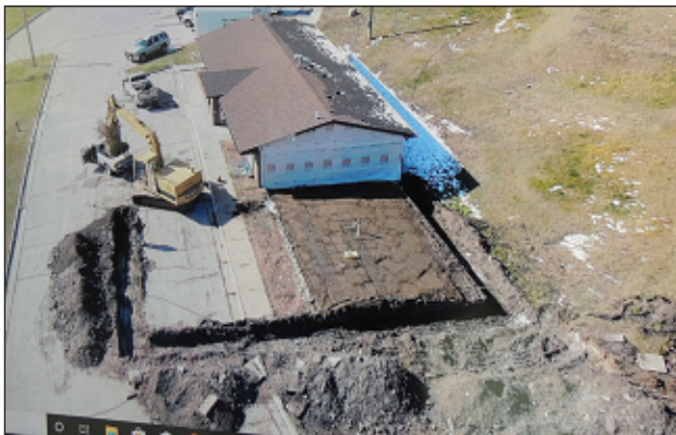
FUTURE SAR GARAGE — An aerial drone shot shows the outline of the new 40'x60' building being constructed on the east side of the present SAR headquarters that will house nearly all of their vehicles and equipment. It will have four bays, two of which will be drive-through.
